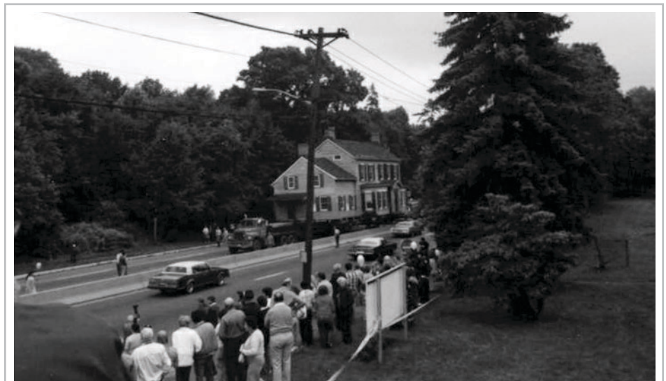
The Hetfield House as it appeared on Saturday, June 29, 1985 traveling westbound on Rt. 22 as it was moved to its current location near the Mountainside Library.
