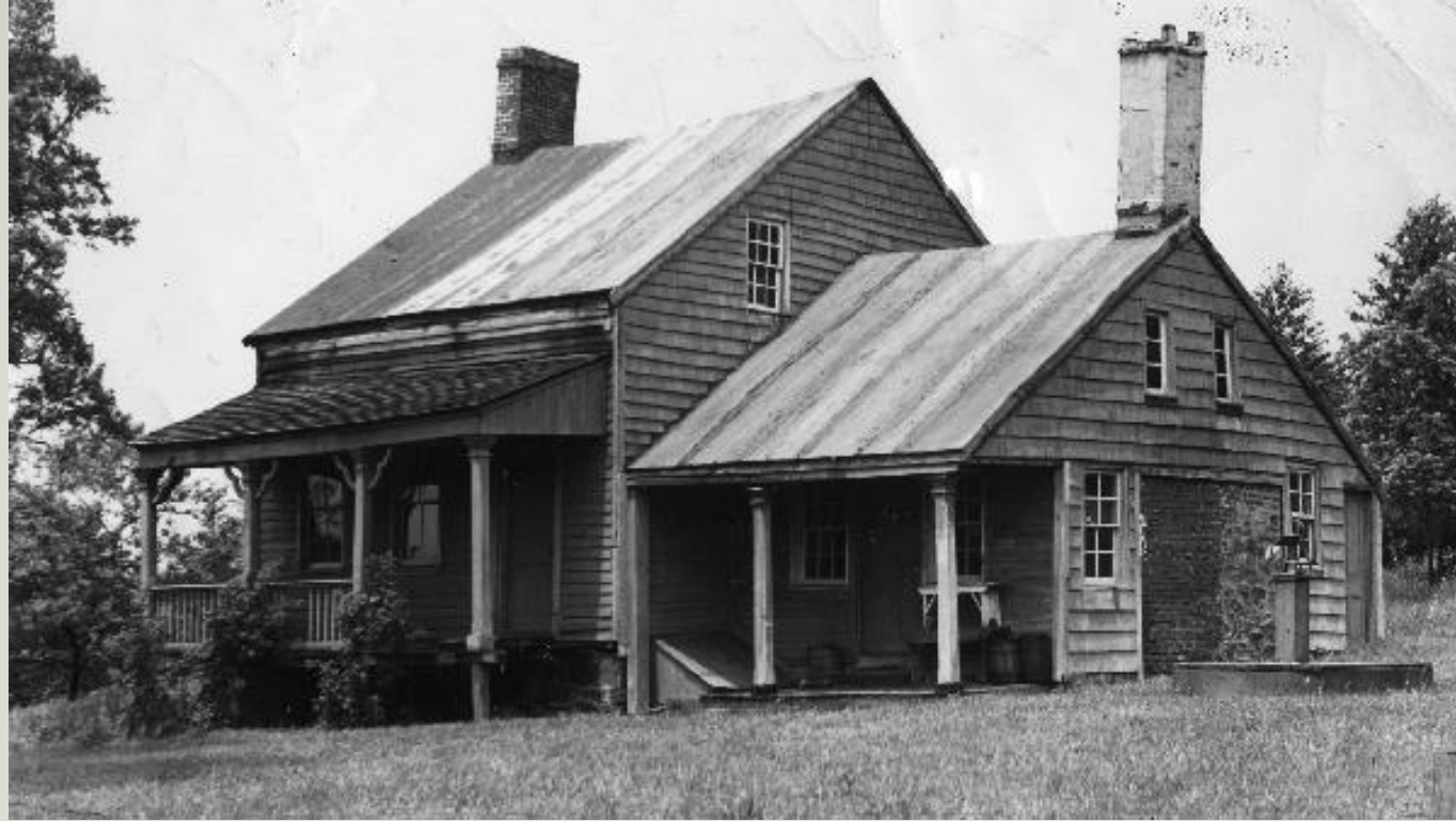
COLLINS HOUSE – BUILT 1790, COLES AVE. NEAR TRAILSIDE, RAZED IN 1960
